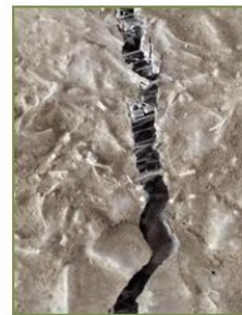
Split Of Ecc Concrete
